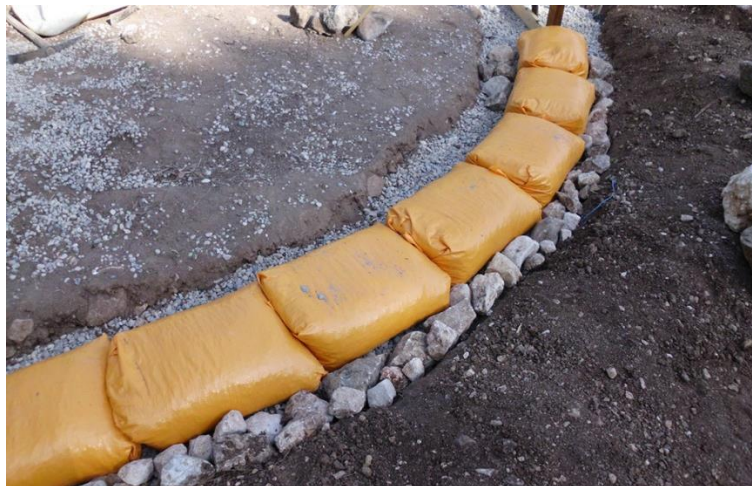
Figure 9: Sandbags of reinforced soil were filled with special fibers that replaced the old straw and mixed with water (Bani Massoud, 2008).
