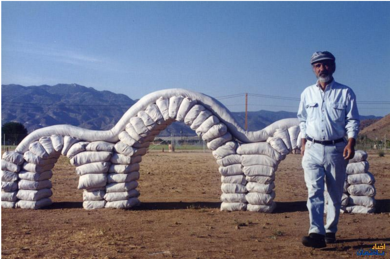
Figure 1: Nader Khalili's photo next to the innovative Super Adobe method inspired by Rumi's poems (Akhbarsakhteman, 2023)
