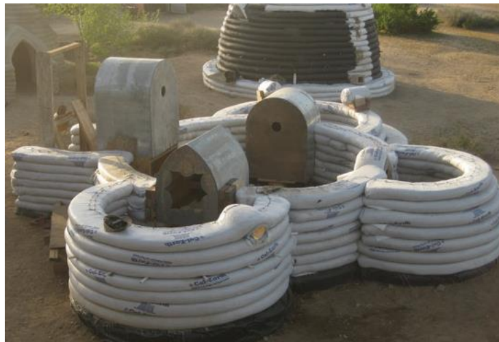
Figure 11: Self-supporting structure resistant to tensile forces "running bond" construction method (Bani Massoud, 2008).
