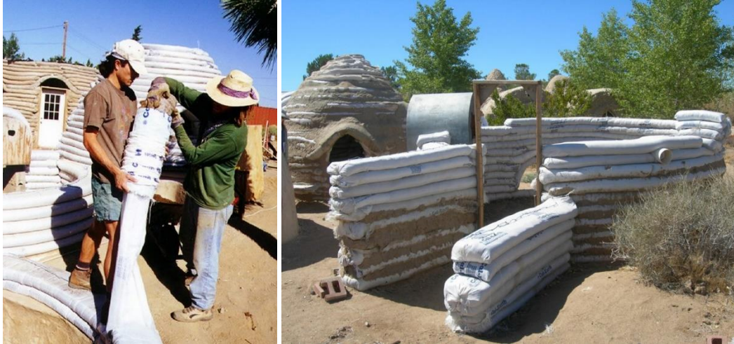
Figure 10: Long strings of clouds of clay have a unique ability to withstand heavy earthquakes (Bani Massoud, 2008).
