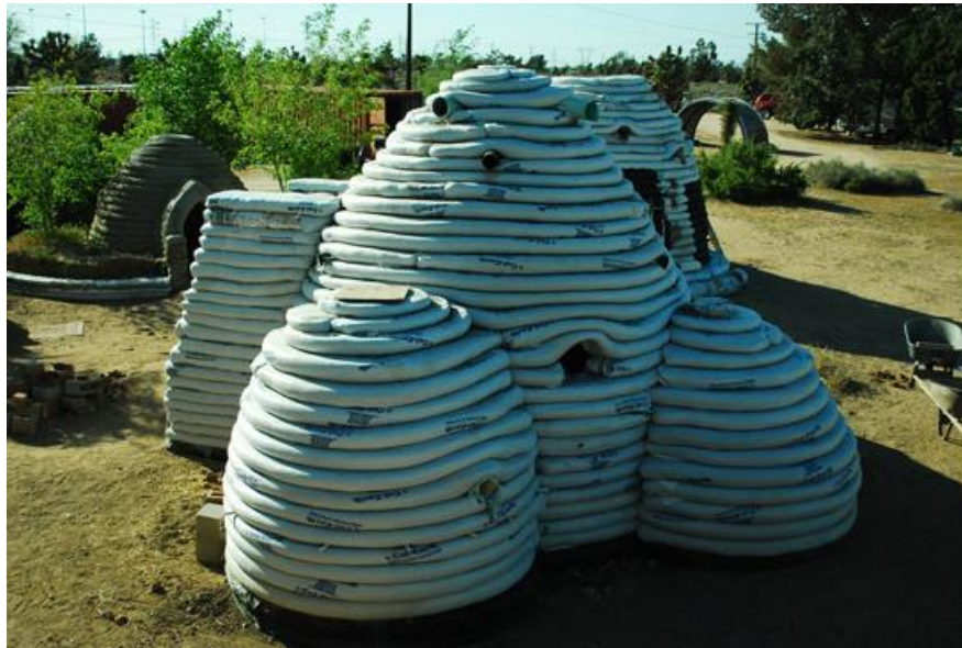
Figure 19: A super adobe system is built using cement and soil, which is low-cost and fast (Naidoo, 2010).
