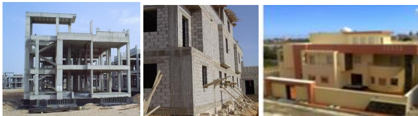
Figure 17 Structure of the contemporary building http://itcadel.gov.ly
