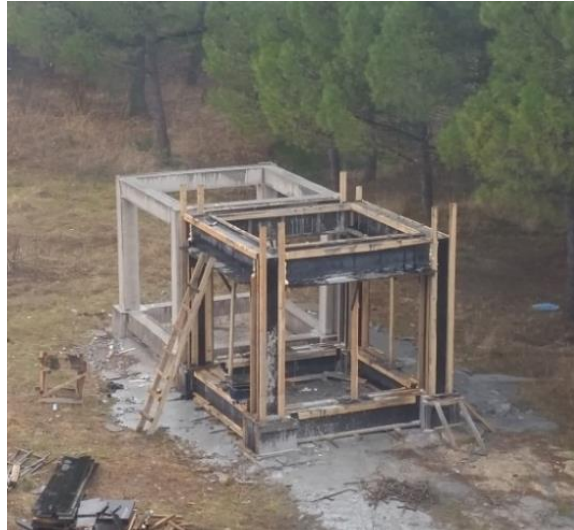
Figure 6. The construction site around two frames
