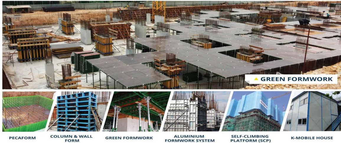
Figure1. Classical kinds of formwork [1]
