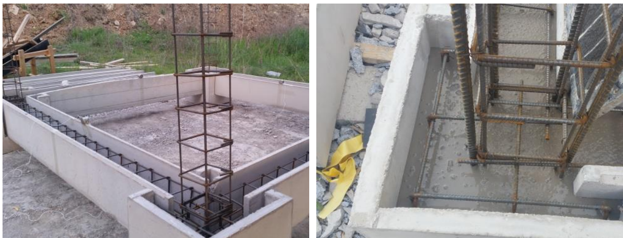
Figure 5. Pouring concrete into the integrated formwork system
