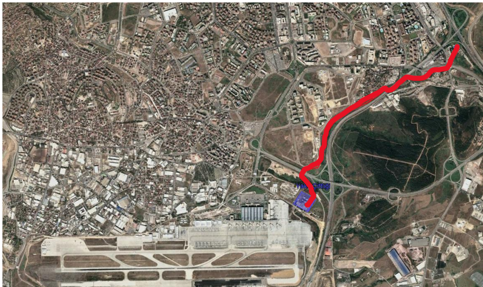
Figure-16. Fuel Supply Pipeline (HEAŞ, 2001)
