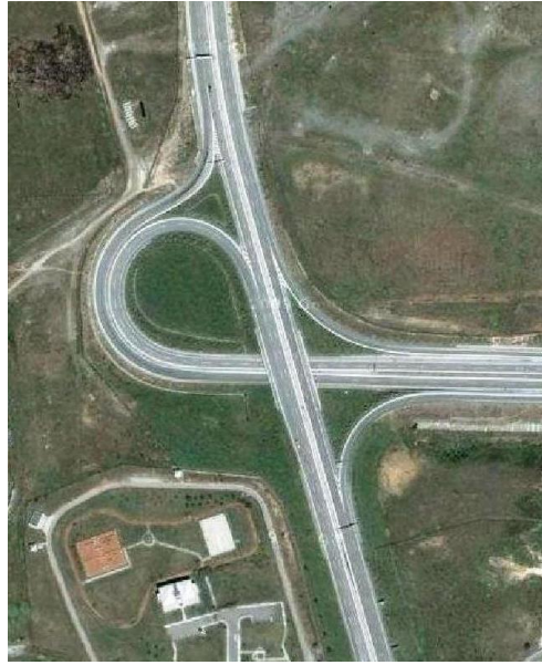
Figure-19. Trumpet Interchange (Google Earth Image, 2023)
