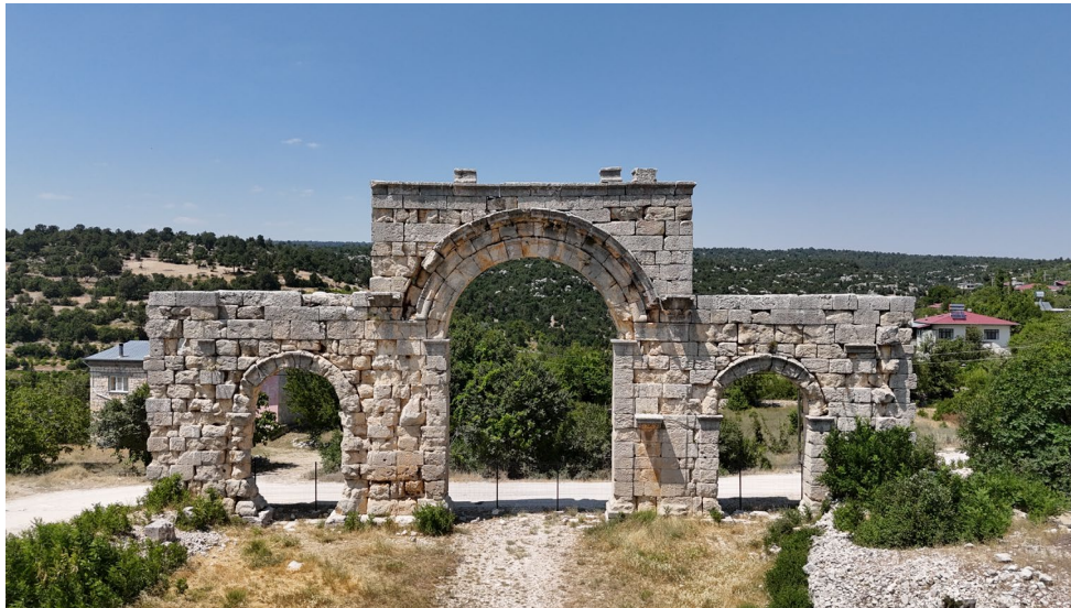
Fig. 4 North City Gate, South Facade
