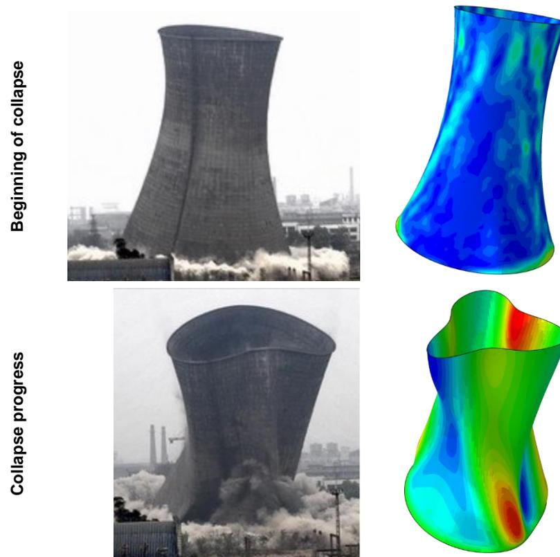
Figure 1. A cooling tower, in a demolition blast in Chengdu, southwest China's Sichuan province: Left, simulation results: Right
