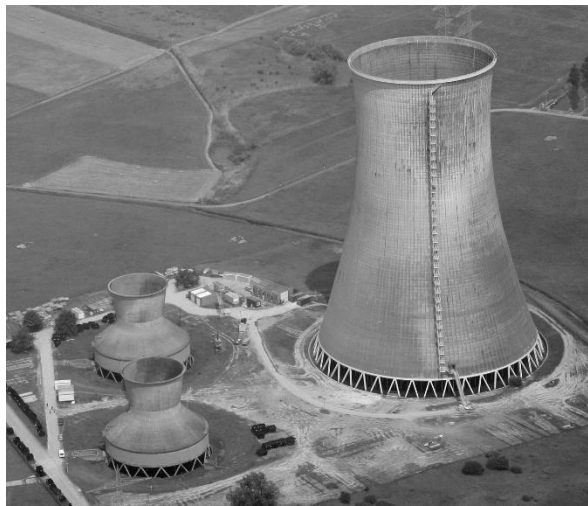
FIG. 4. Industrial cooling tower at a power station
