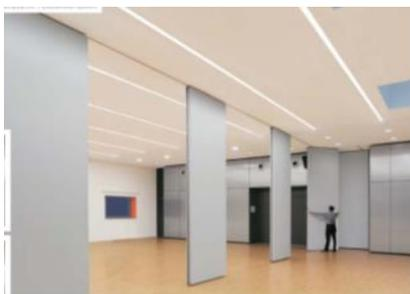
*Figure 8. Sliding folding panel wall [7]*
