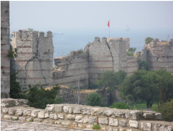
Photo 3. The land walls of Istanbul suffered severely from natural disasters especially from earthquakes. (M.Somuncu)
