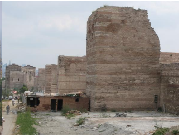
Photo 4. Part of the land walls under restoration work. (M.Somuncu)
