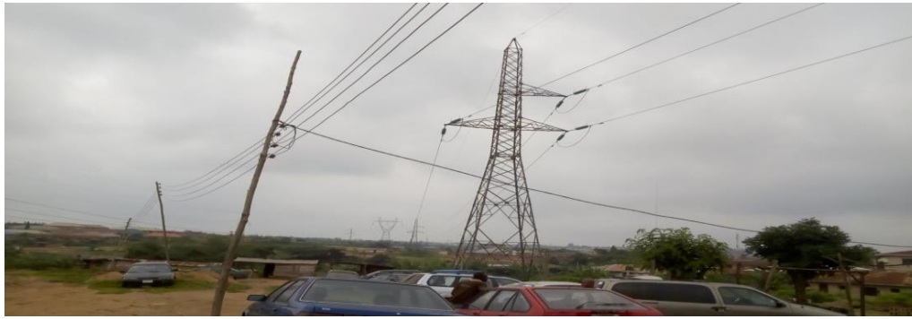
Figure 1. Automobile mechanical workshop under 330/220 kVA power transmission line in Osogbo
