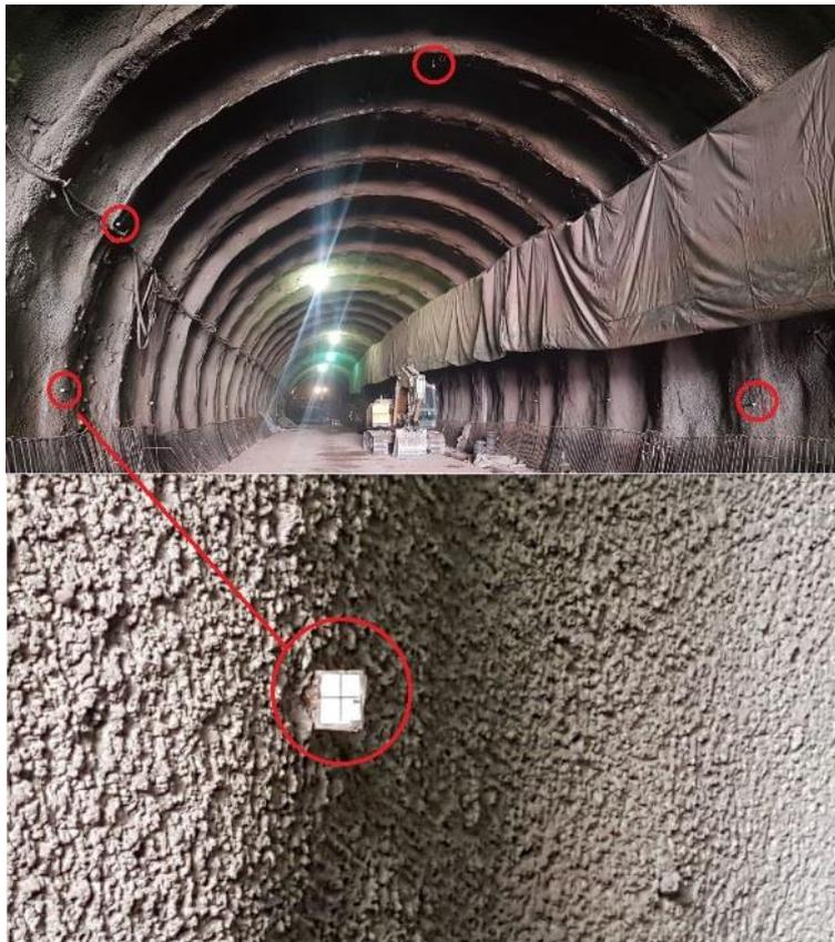
Figure 6. Tunnel deformation target.
