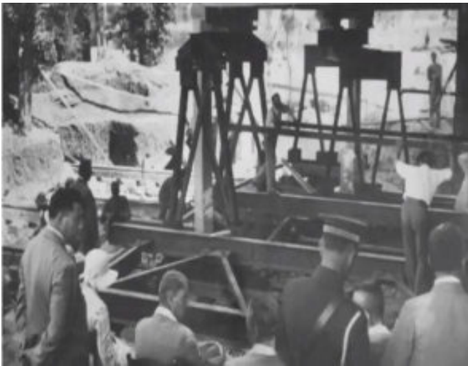
Photo. 3 and 4: The Relocation Operations of The Moving House Photo source:Engin Çakır;Dergibursa.com.tr; http://www.dergibursa.com.tr/doga-sevgisinin-kosk-hali-yuruyen-kosk/
