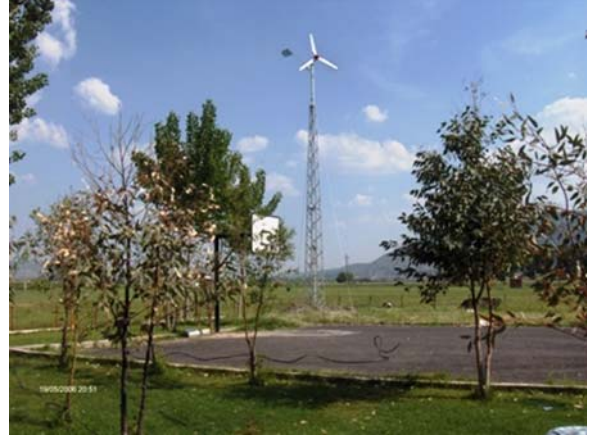
Şekil 2. Kurulu sistem (The constructed system)
