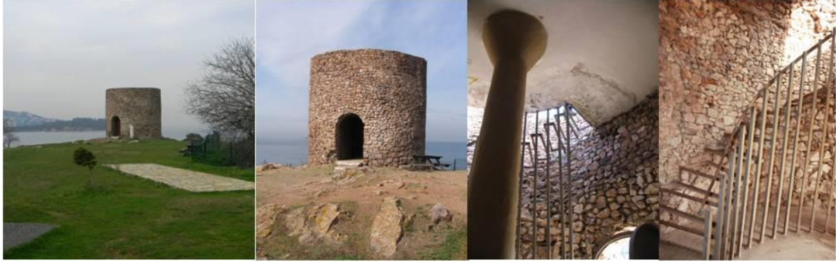
Figure 2 Current state of the mill (Kıraç,B., Töre,T., 2014)
