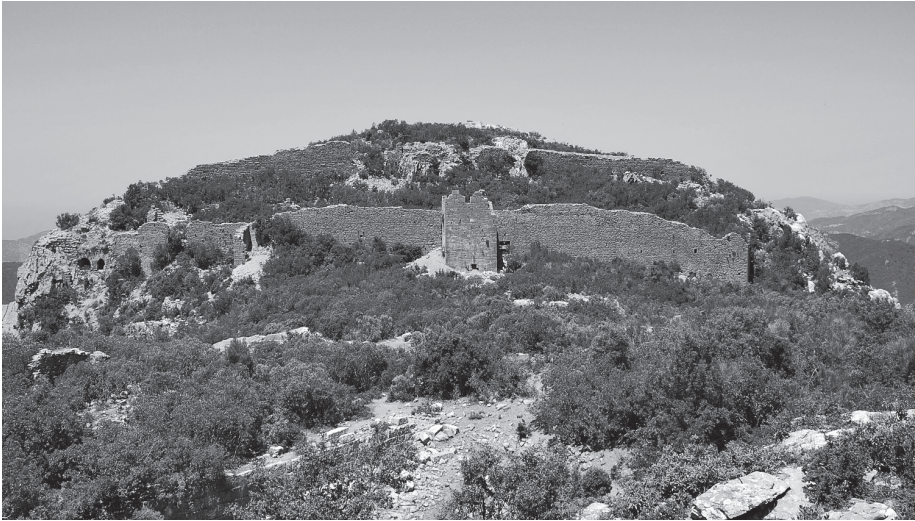
Fig. 7. Lamos, acropolis fortifications, from east
