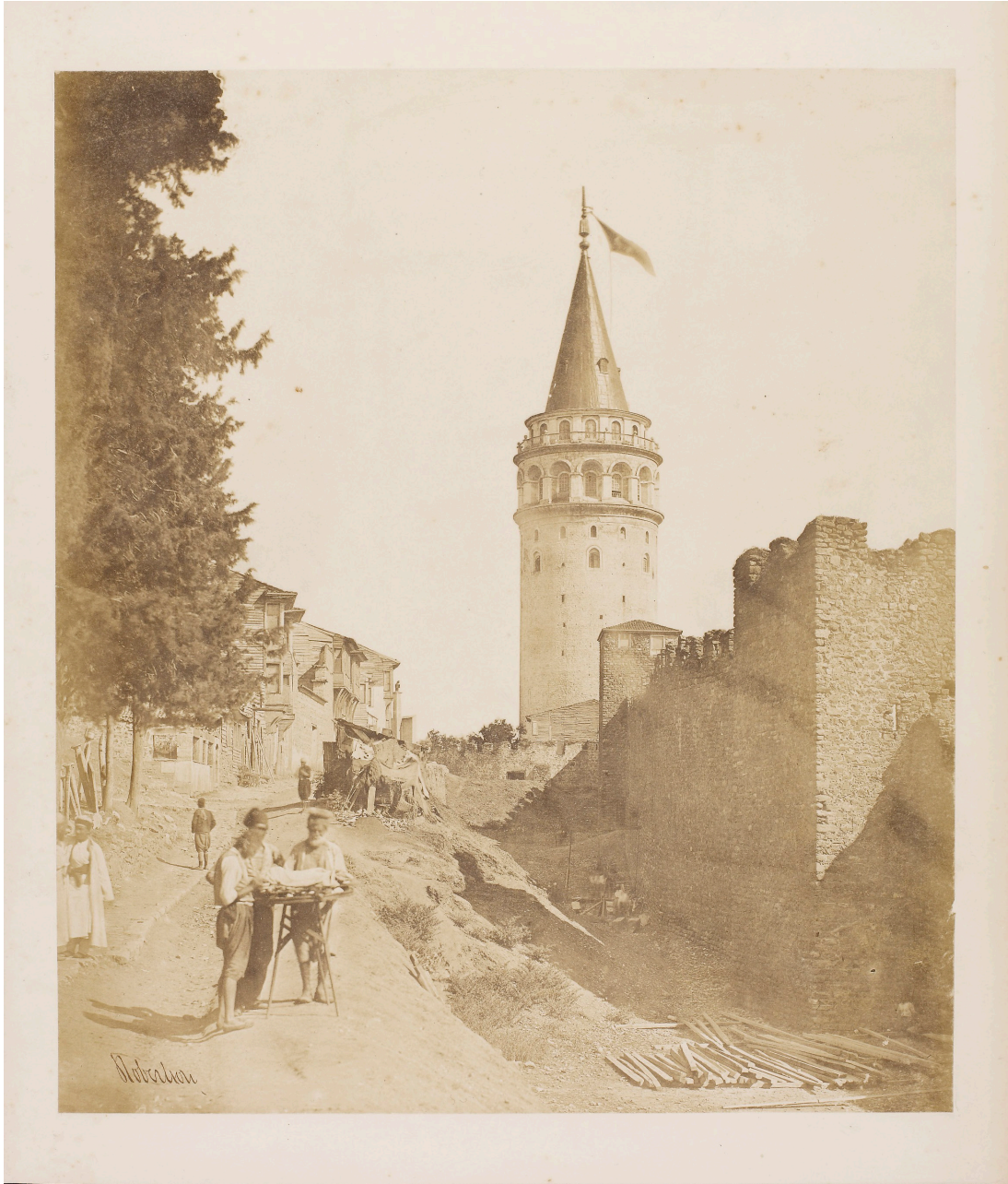
Figure 4. The walls of Galata before the demolition.
