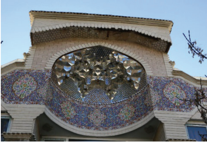
Fig. 2. Muqarnas, mirrored decorations, and Haft rang tiles in the exterior view of a house in Jomhoori Eslami ST. In Shiraz built in the Pahlavi era (Photo by Dordaneh Mohammadi, 2016)
