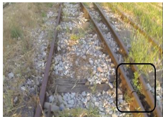
Figure 4.3. Control of rail fasteners
