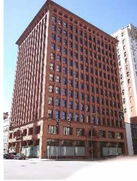
Şekil 8. The Puridential (Guaranty) Building ( Steven H. Photo Systems, 2012 )
