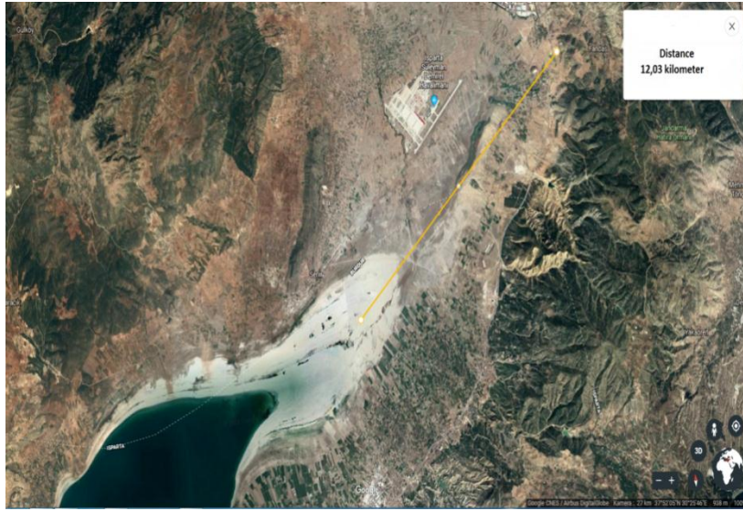
Figure 4. The location and distance of Gökçekuyu Solar Power Plant
