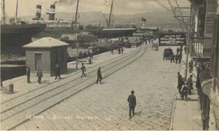
Figure 7. Train Lines of Kordon. Abdullah Erek Donation Fund, Ahmet Piriştina City Archive and Museum.
