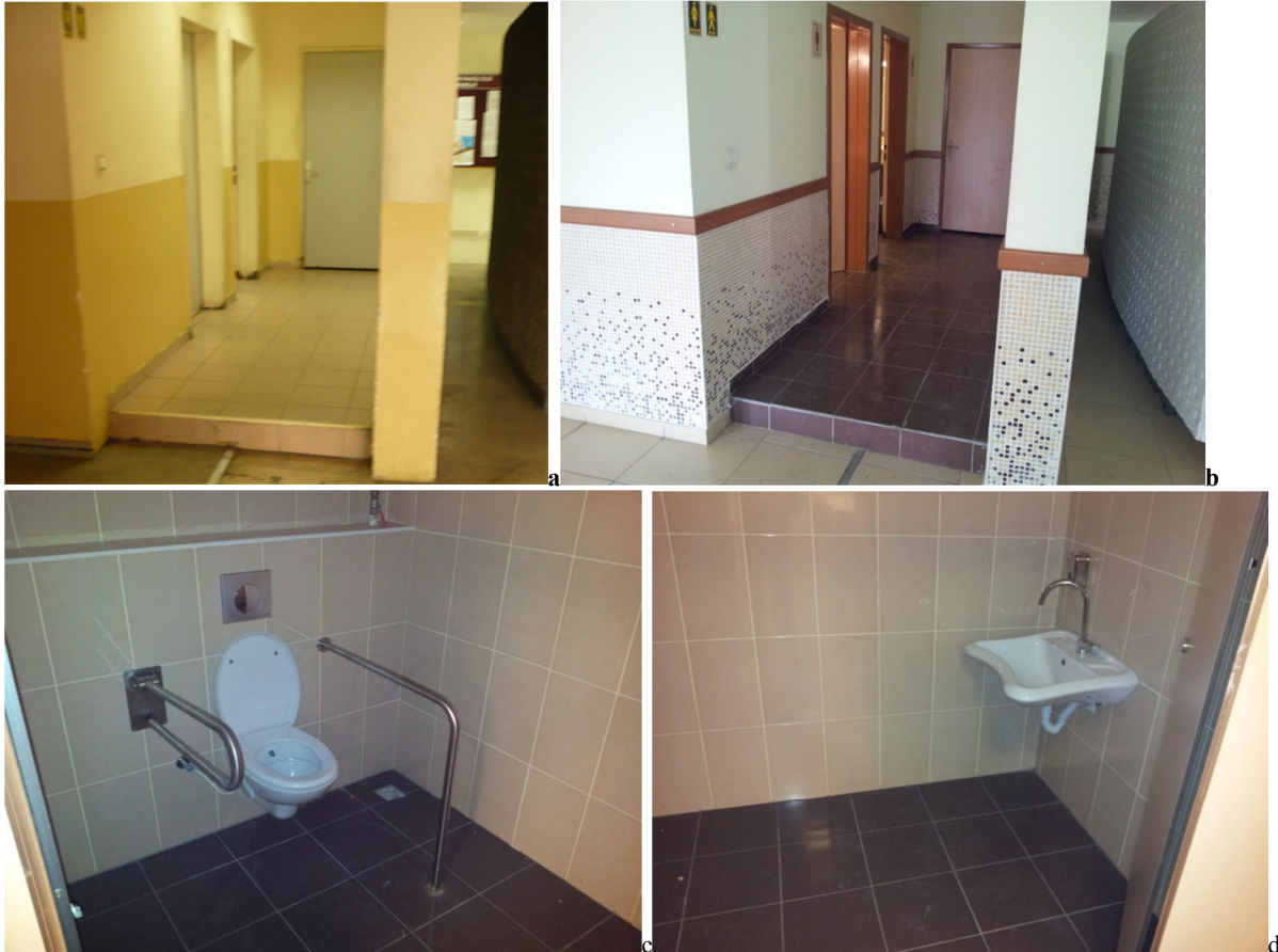
Figure 11: Water Closets (Ground Floor) a:2011, b: 2012, c: 2012, d: 2012
