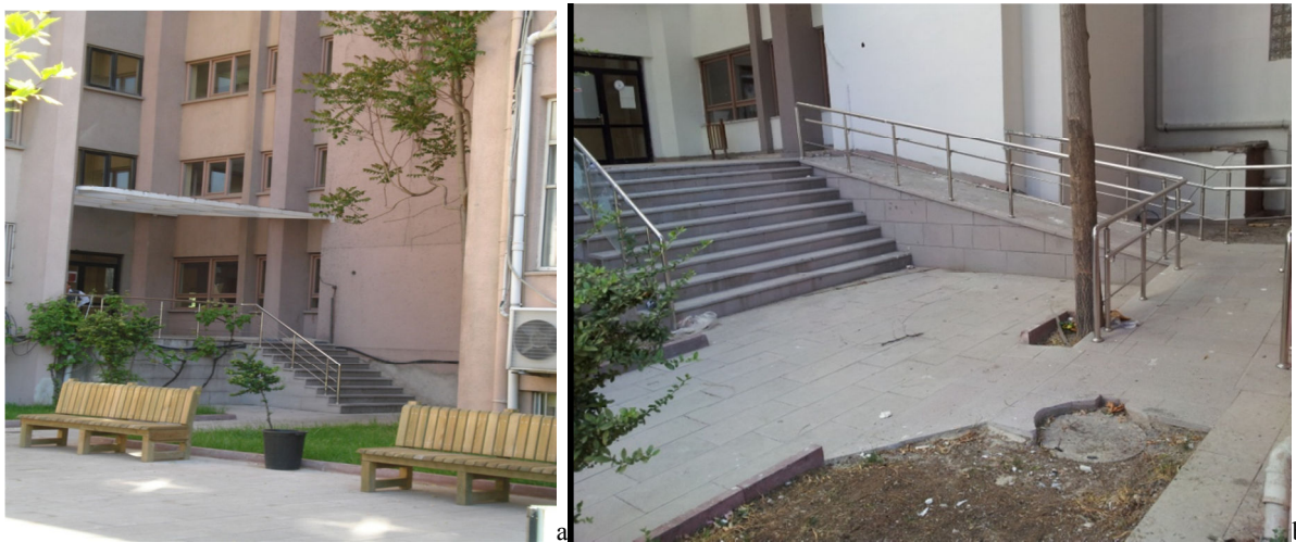
Figure 5 Sec. Building Entrance (to External Yard) a:2011, b:2012
