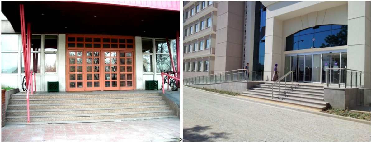
Figure 3. Primary Building Entrance (to-OPA-Site Ent-1) a: 2011, b: 2012
