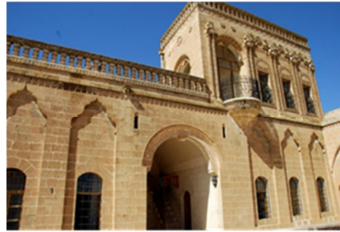
Figure 1. Traditional Midyat House [15]
