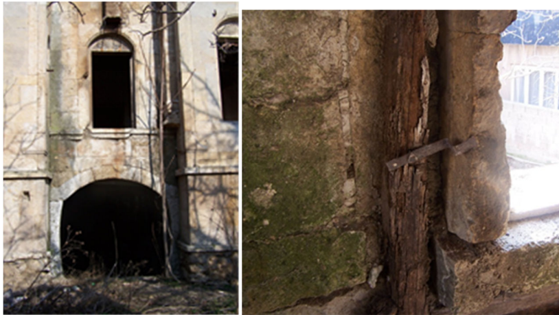
Figure 20. Stone facing on the timber frame wall [22]
