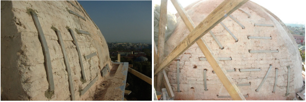
Fig. 5 - Cap view from the top of the main piers 6 and 7 [34, 35]
