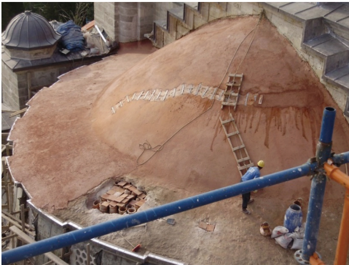
Fig. 4b - Side dome view around the station 4 from outside [34]
