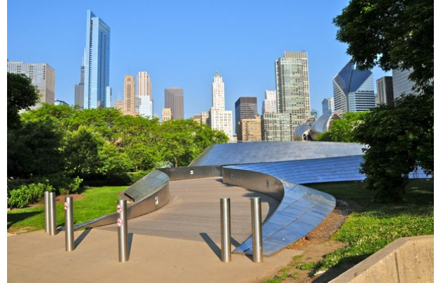
Şekil 26. Millennium Park BP Pedestrian Bridge, Chicago, ABD
