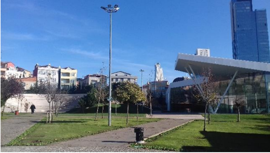
Figure 6 and 7. Steel structure of new social centre and health centre, make habitants feel like it can be moved easily, in case there will be urban transformation, they can be moved as well. Photo by the author.
