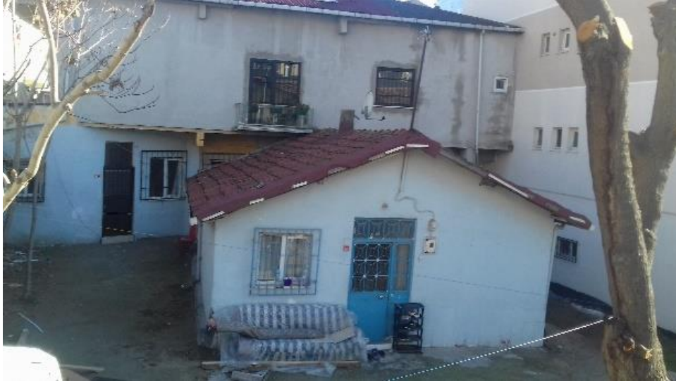
Figure 3. Layers of housing activities. 70s building that was planned and shared equally, with garden voids, and behind 80s building. Photo by the author.
