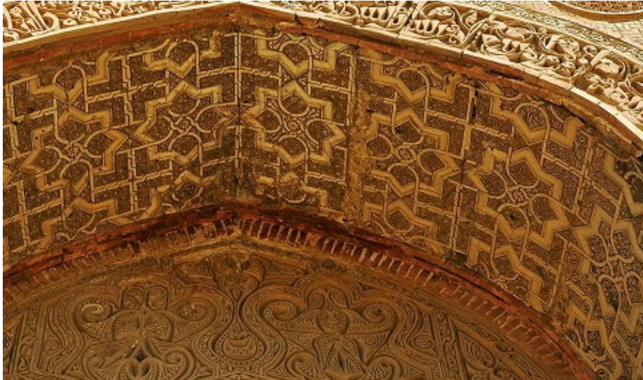
Fig. 4. This same design, bound together by a layer of “inter-lace,” on the underside of the arch of the portal of the 1152 Karakhanid Jālāl ad-Dīn Hūseyin Turbé, Özkent, (modern Kirgizistan) 13 .
