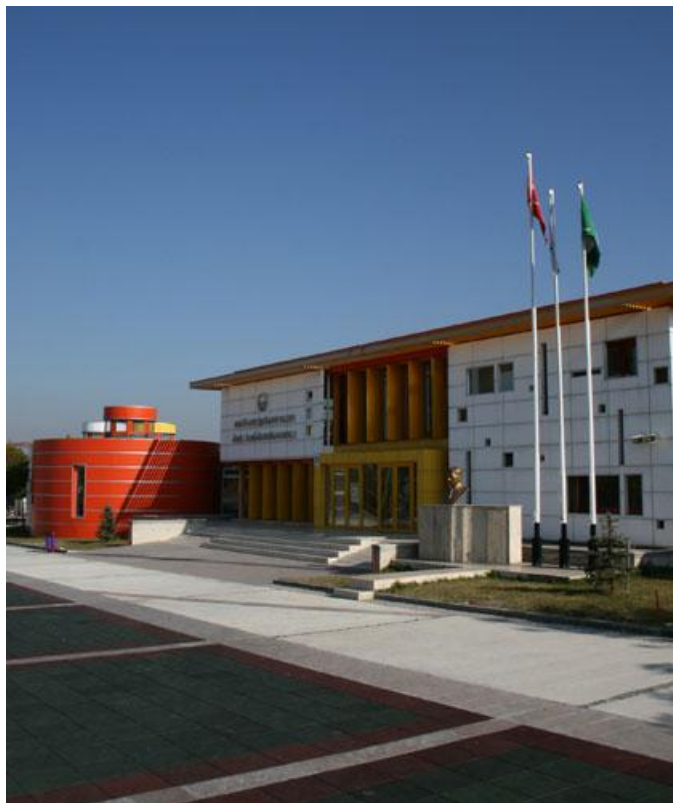
Figure 2 Private Primary School building
