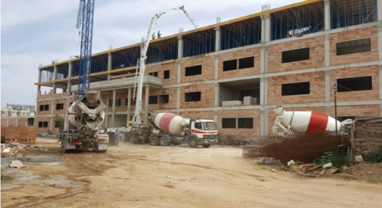
Figure 4 - View of the Main Access Point
