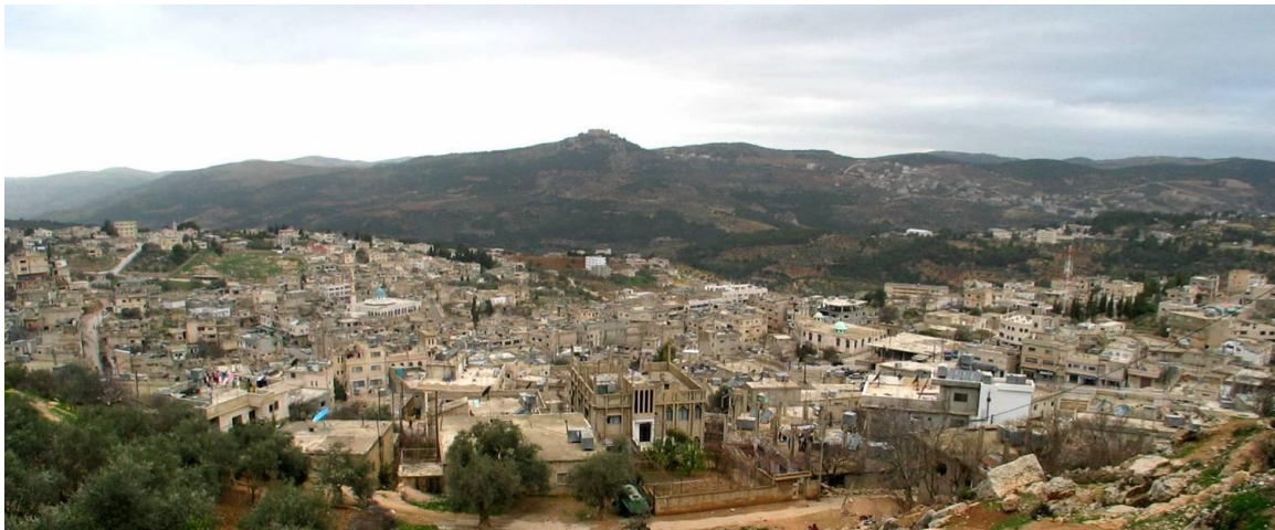
Figure 2 Anjara general view
