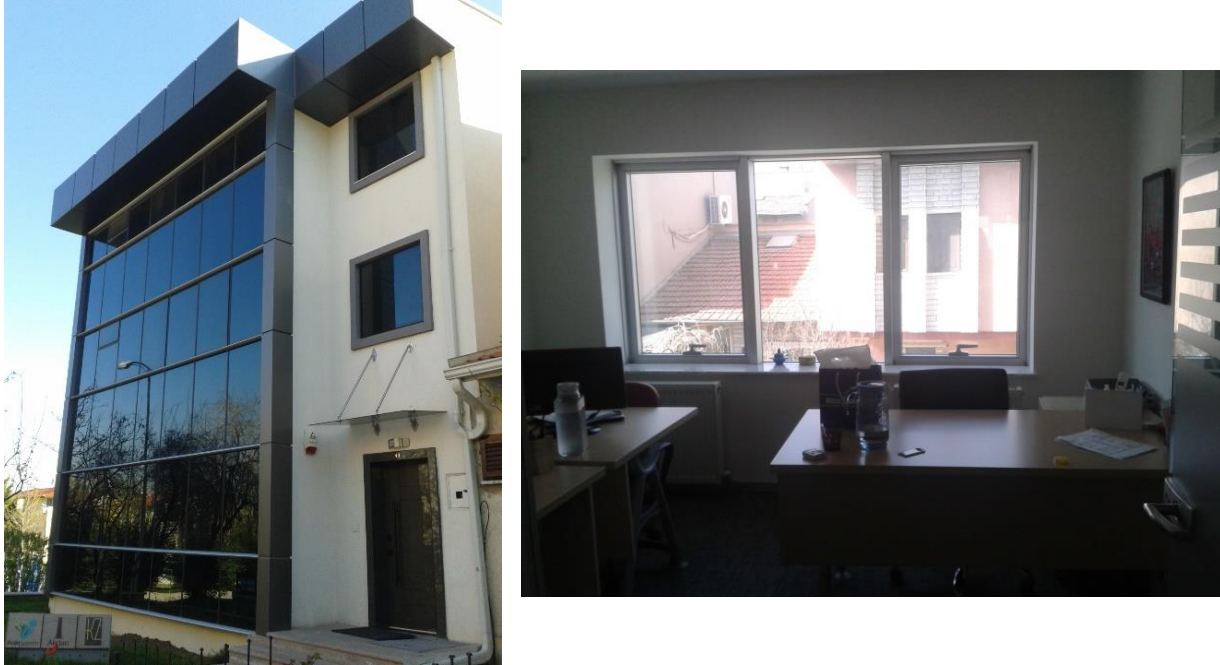
Figure 2 At left Building 1 exterior picture that examinations were mainly went on. Photo was shot at 21st April, 2015. At right, an interior image of Building 1 showing the exterior walls adjacent to the curtain wall. The photo was shot at 27th April, 2015.
