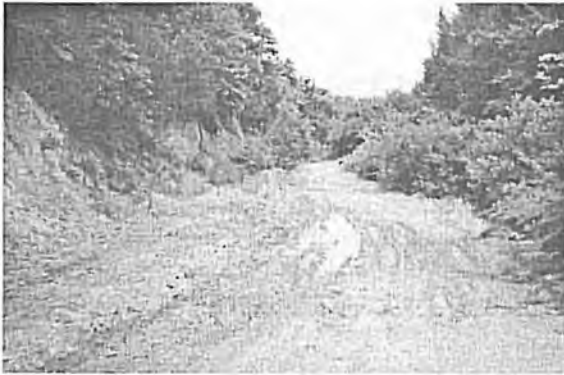
Figure 3. The conditions of 02 code forest road, ditch, and roadbed prior to pavement activities (Photo: T.Ozturk)
