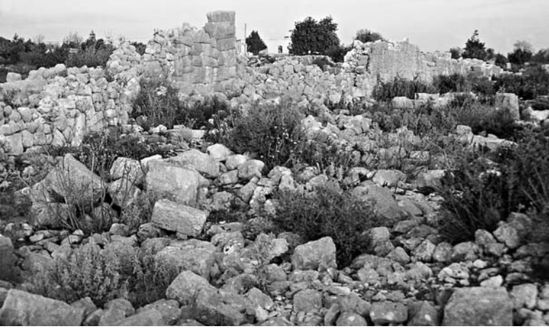
Fig. 2 Pashı, Fortification Wall
