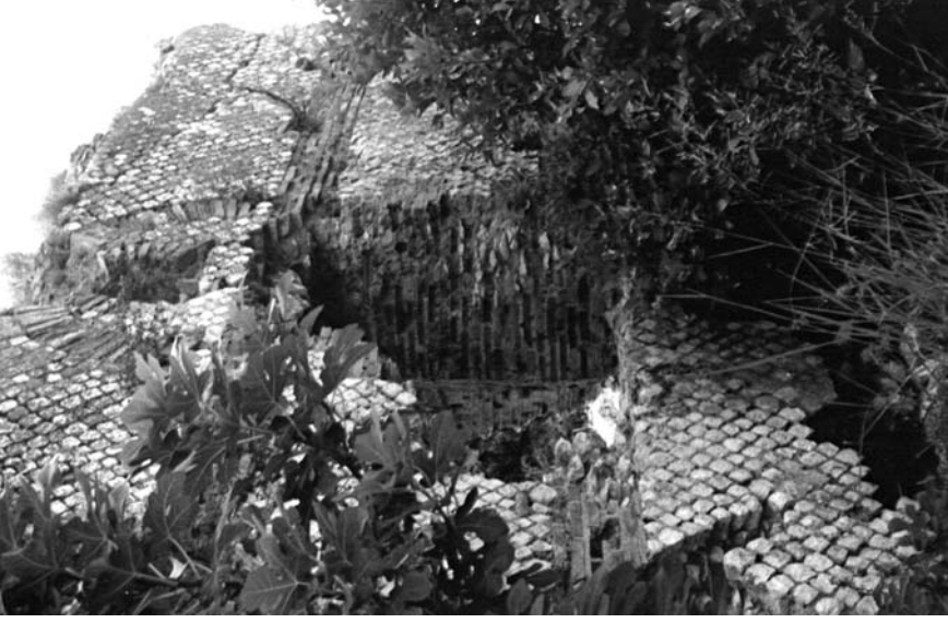
Fig. 17 Roman Baths in Elaiussa Sebaste (Ayaş), opus reticulatum construction (photo: Yegül)
