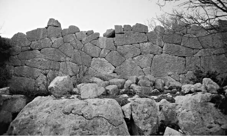
Fig. 14 Veyselli, Fortification Wall
