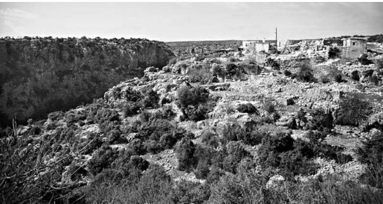
Fig. 4 Hüseyinler, Location and Tower (?)
