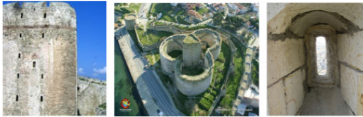
Photo 2a, 2b, 2c: Kilitbahir Castel , Dardanelle, TURKEY
