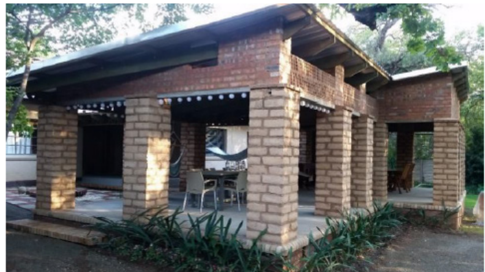
Figures 3 & 4. On-site stabilised earth block production of a demonstration building project constructed in a residential area of Bloemfontein, South Africa (2016)
