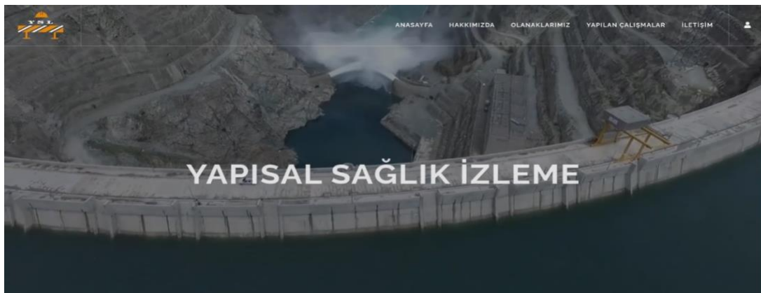
Figure 5. Structural Health Monitoring website.
