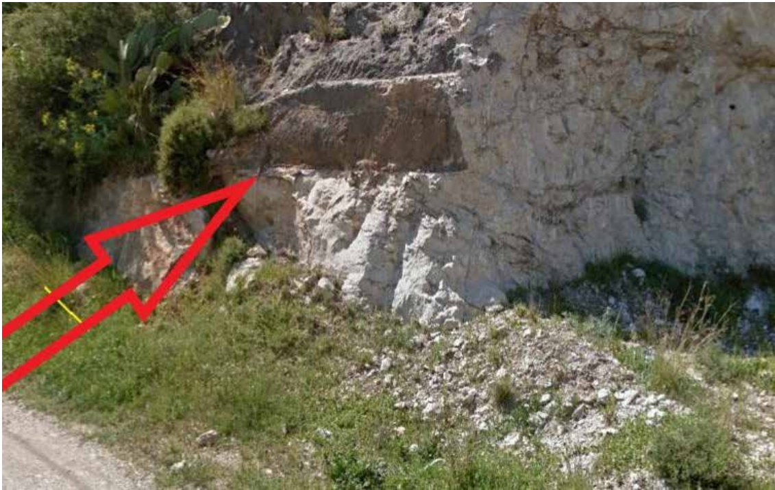
Figure 7: Remains of the First (Roman) Waterway (Ankara District) Mahalleşi
