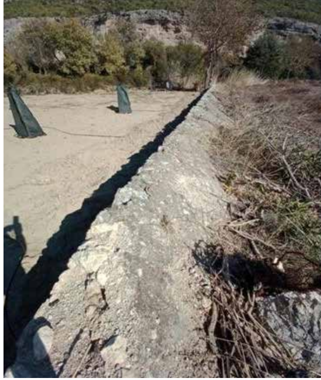
Figure 15: Gavurun Dam (Gavurun Barajı)
