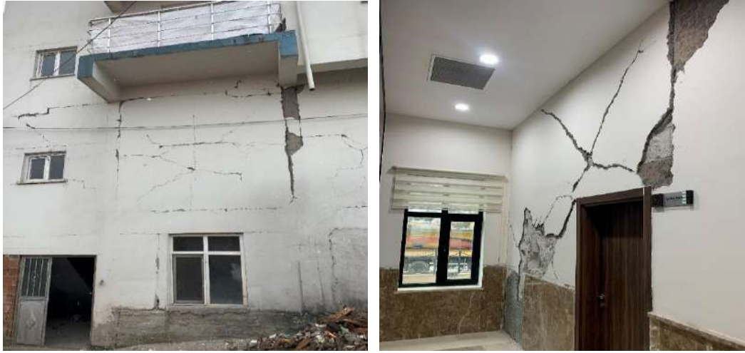
Figure 11 In-plane damage
