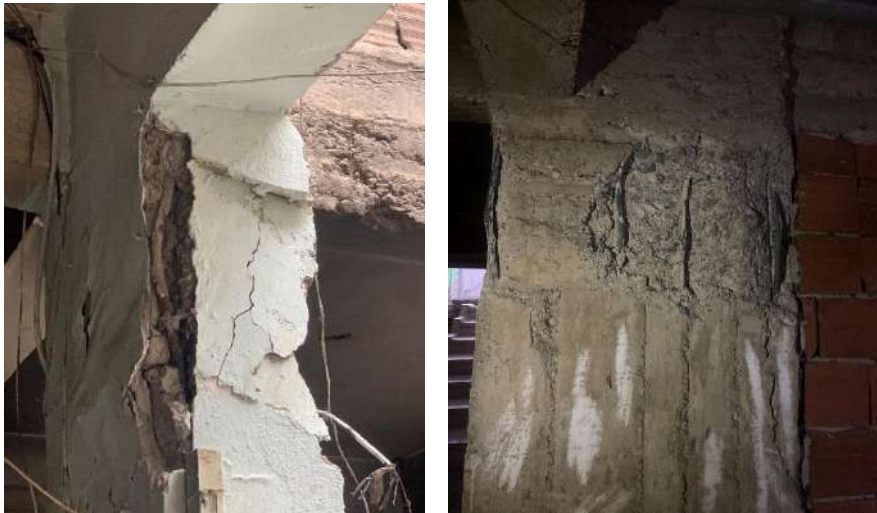
Figure 8 Buckling longitudinal reinforcement bars of damaged column due to insufficient transverse reinforcement
