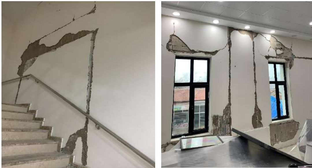
Figure 13 Disconnection of infill wall from the frame
