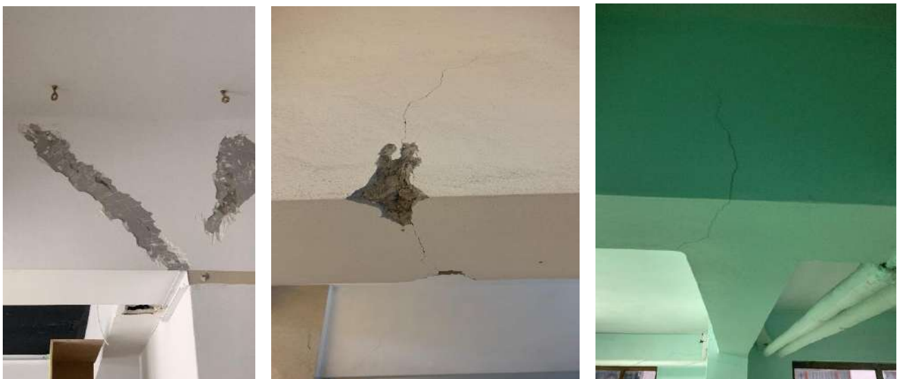
Figure 9 Beam damages
