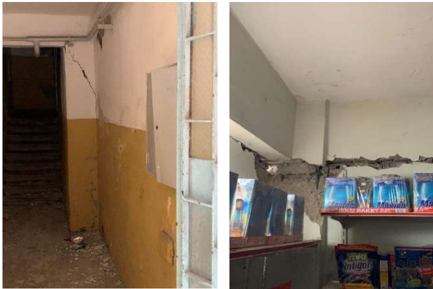
Figure 10 Strong beam–weak column
