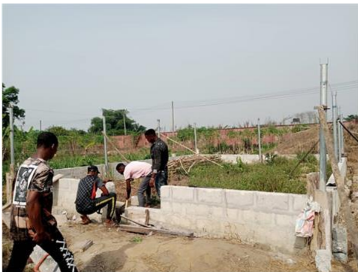
Figure 2. A typical building construction site.
