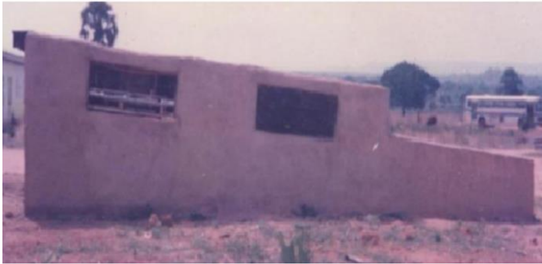
Figure 18. Solar dryer constructed with mud solar thermal collector (Eke, 2014).
