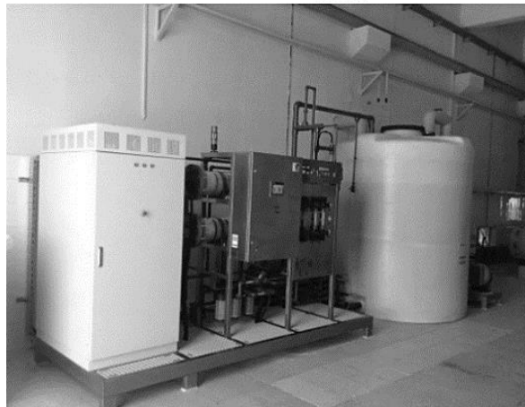
Figure 4. The equipment of on-site sodium hypochlorite generation system
