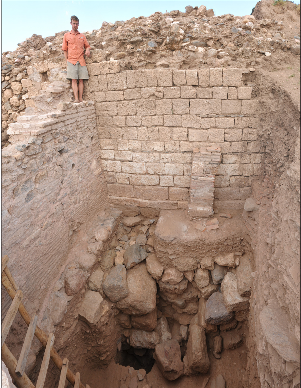
Figure 7: Field 49, western terrace wall showing upper limestone section and lower boulder wall, with archaeologist Will Bruce.
