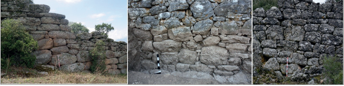
Figür 25. Harpasa, Kaunos ve Keraitai duvar tipleri / Harpasa, Kaunos and Ceraitai masonry types.
