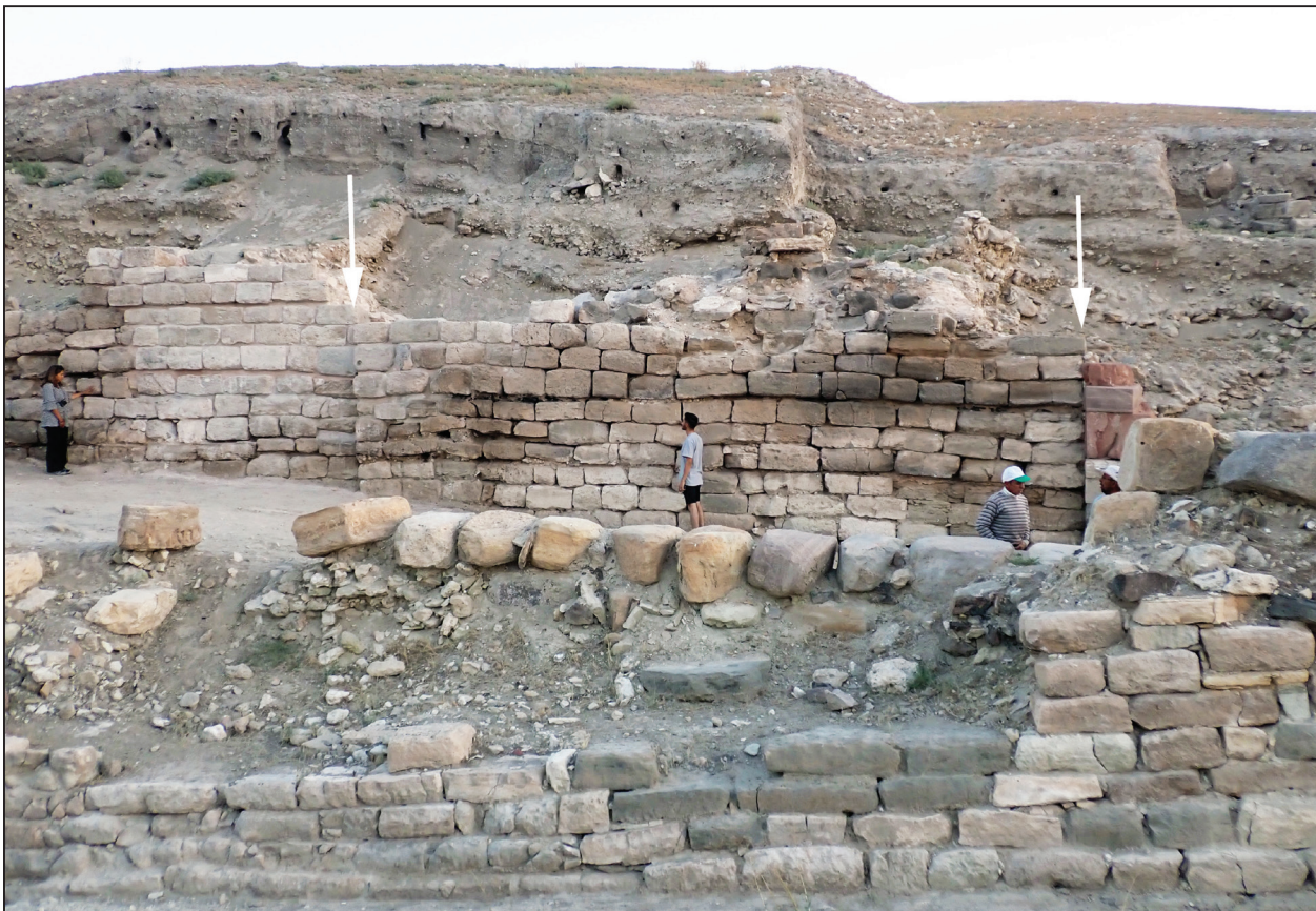
Fig. 9. The newly conserved north wall of the South Gate (9th century B.C.). The arrows indicate vertical offsets in the wall. A glacis, or stepped terrace wall, is in the foreground. (Photo by Brian Rose; courtesy Penn Museum, Gordion Project Archives.)
