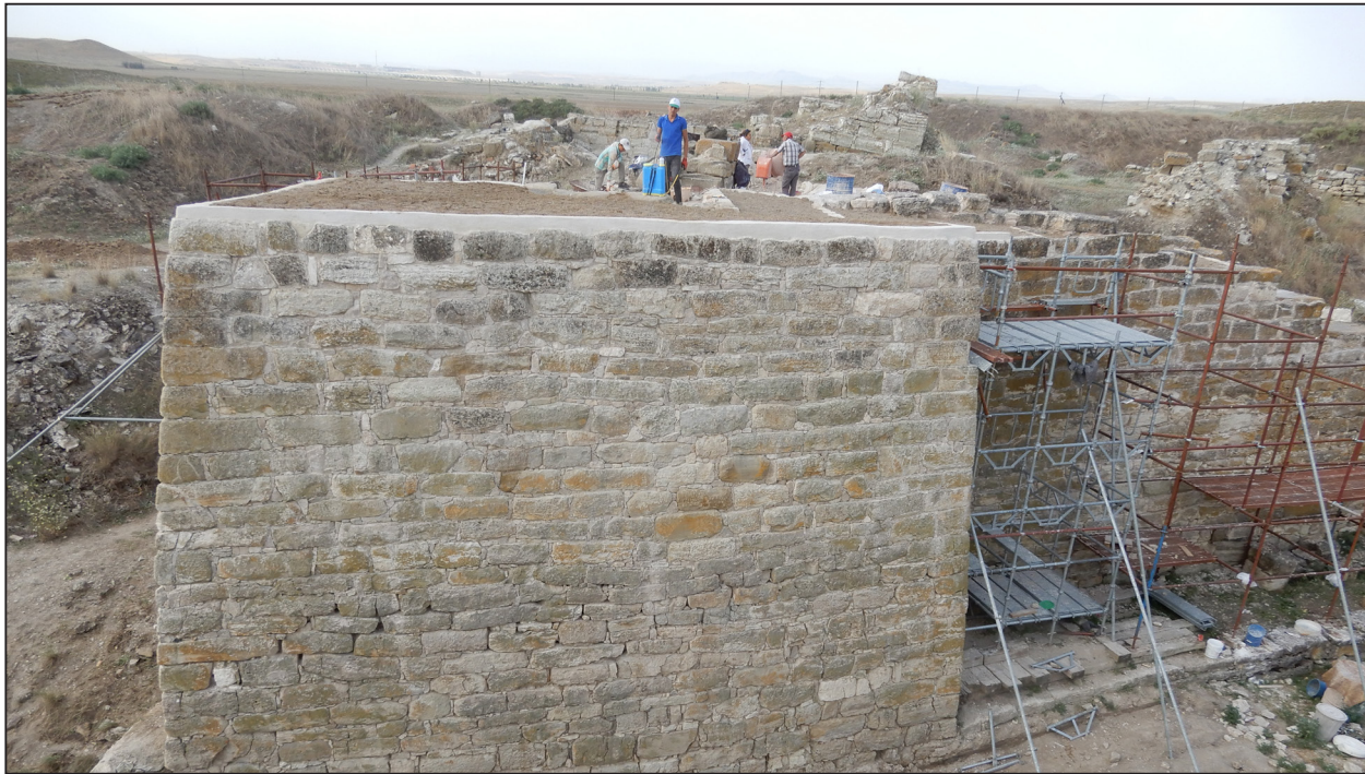
Fig. 6. East Citadel Gate: north face of the South Bastion following the installation of the soft-cap. (Photo by Brian Rose; courtesy Penn Museum, Gordion Project Archives.)
