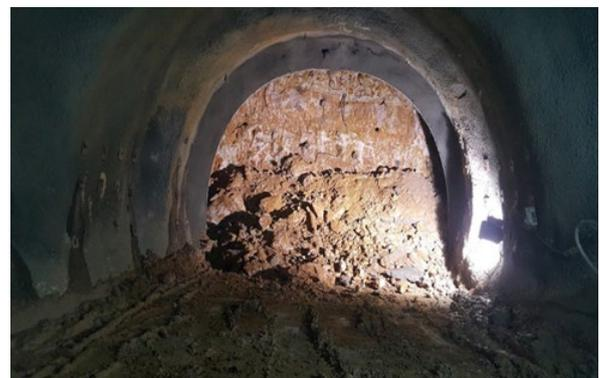
Figure 4. Excavation surface and lining of surrounding rock.
