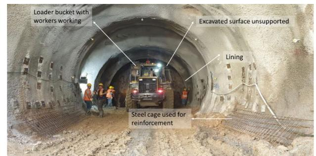
Figure 5. Working environment in the tunnel.
