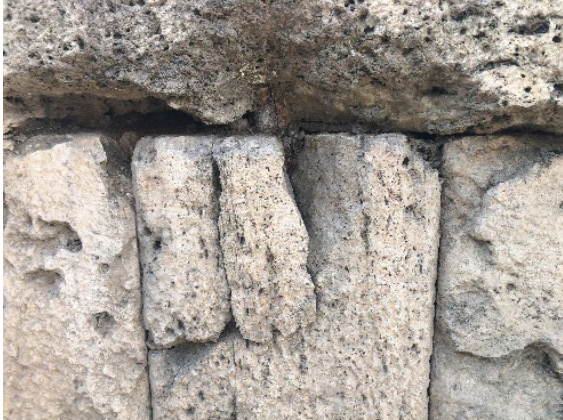
Figure 17 Iron clamp in balustrade
