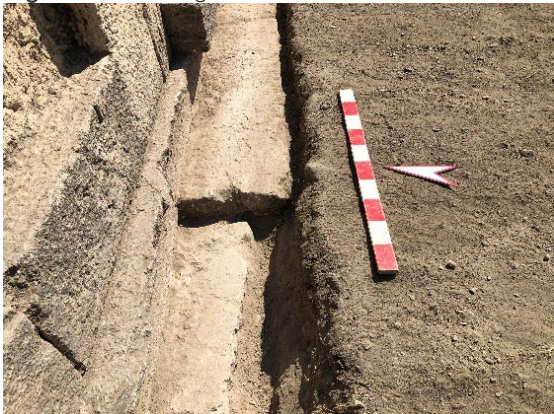
Figure 13 Blockage in front of the stadium
