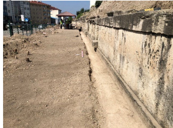
Figure 12 Blockage in front of the stadium
