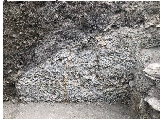
Figure 16 Blockage filler behind balustrade
