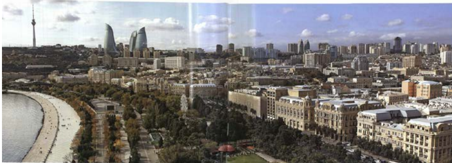
Picture 12: Buildings in Baku where Aglay stone was used. 86
