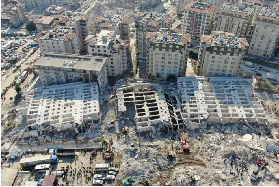
Şekil 1. 6 Şubat depremleri sonrası Hatay’da yıkılan yapı denetimli bir yapı (The building that collapsed in Hatay after the February 6 earthquakes was a controlled structure) [17]
