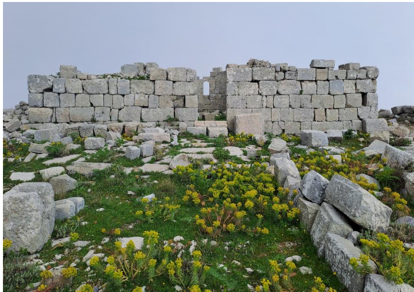
Figure 5: West exterior facade (M. Kaya, 2024)
