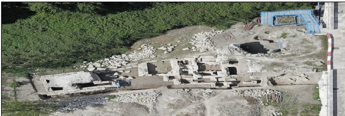
Figure 5. A view of the bridge's vaulted structure, bathhouse, and cistern sections (ANB, 2025).
