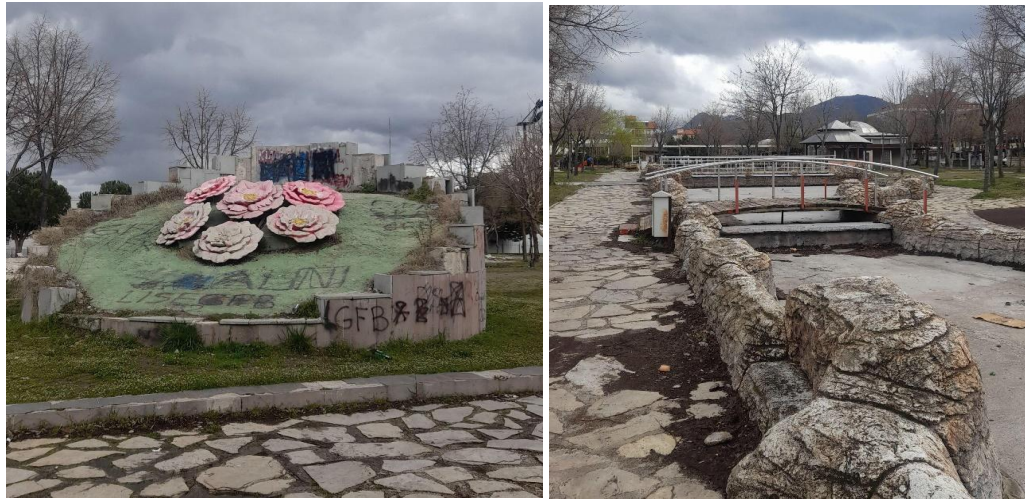
Figure 6. Deteriorated spatial elements in Böcüzade Park (Gedik, 2026)
