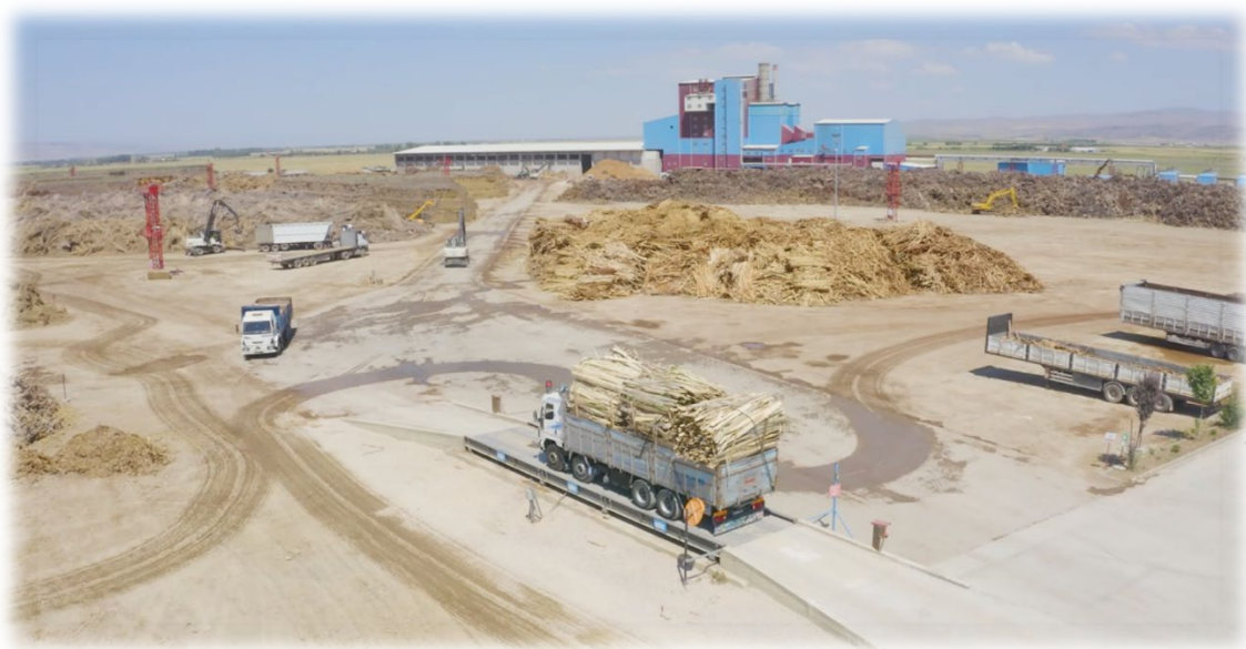
Figure 1. Afyonkarahisar Eber Biomass Power Plant (27 MWe, Çay district)
